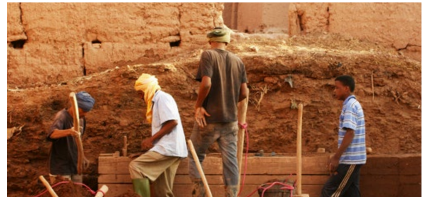
Construction of a rammed earth wall
