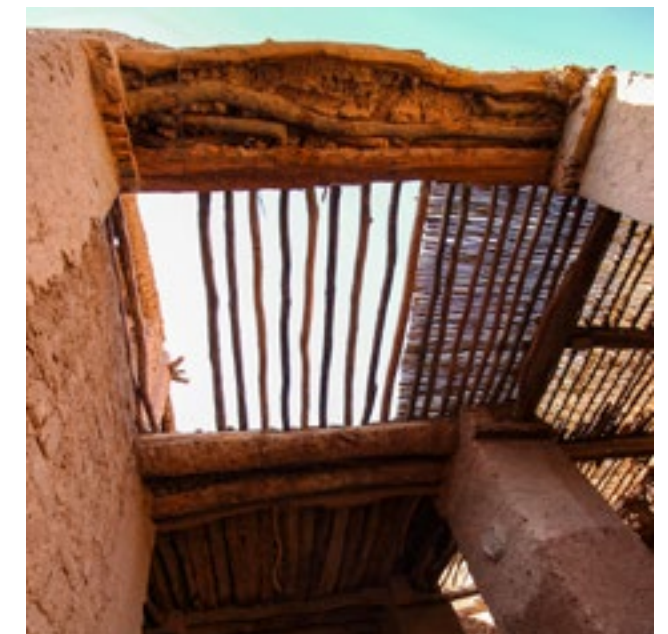
Roof construction with tamarisk branches and reed mats
