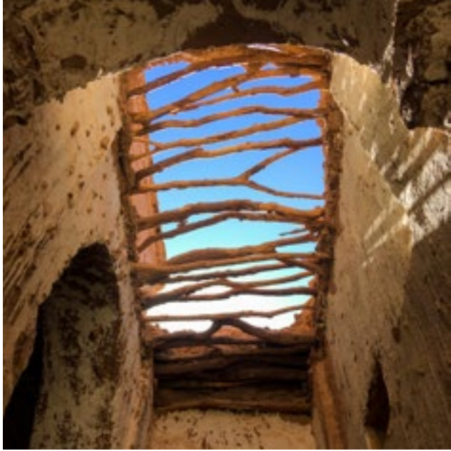
Timber roof of the marabout before restoration
