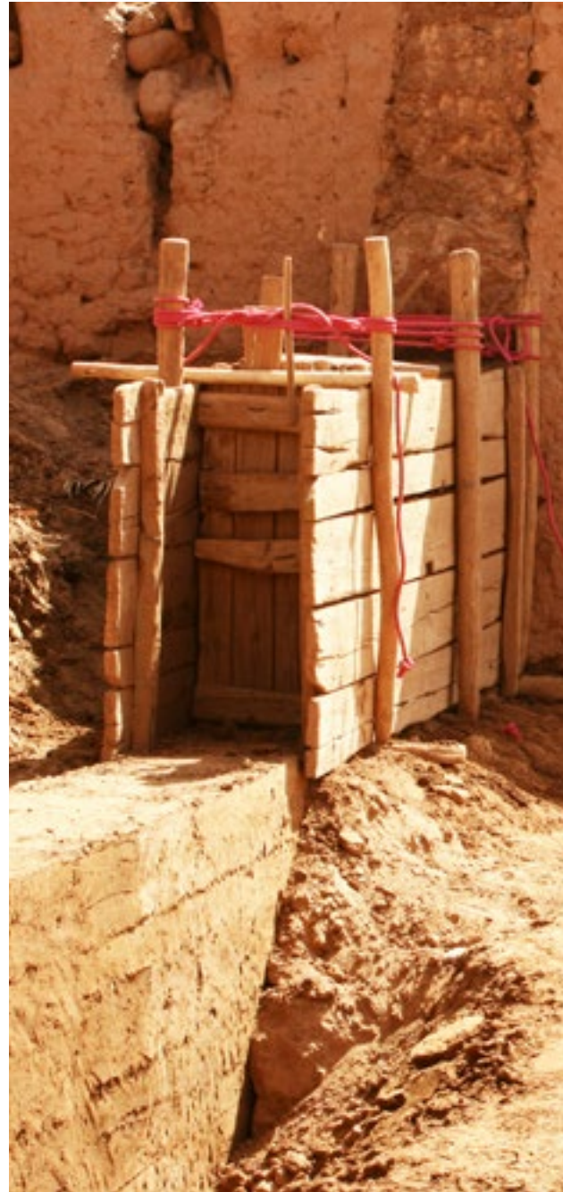
Rammed earth wall and wooden formwork
